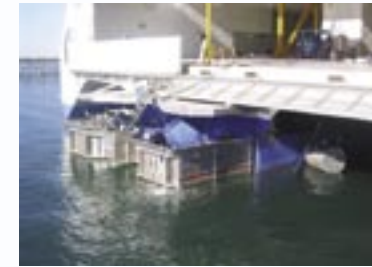
• The cofferdam pumped dry and in position under the vessel.
