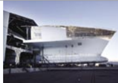
The bow module is moved and attached to the main structure
