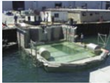
• Cofferdam in position ready for use.
