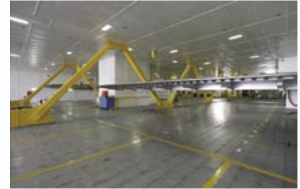
• Vehicle deck showing mezzanine levels enabling mixed loading of cars and trucks/buses for flexible payload.
